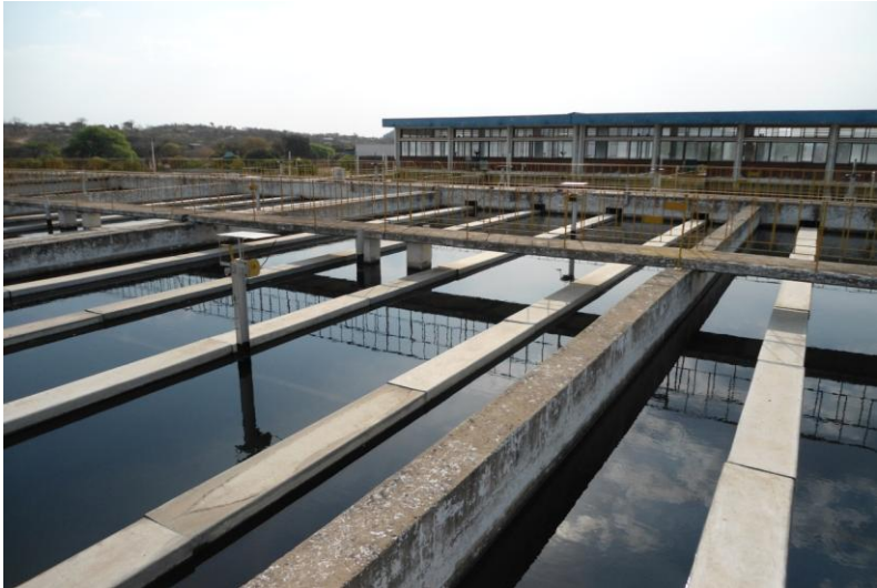
Water Treatment Facility in Lusaka
