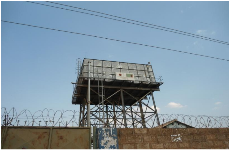
Water Supply Project in George Compound, Lusaka
