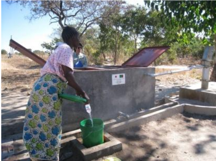
Ground Water Project in Luapula Province
